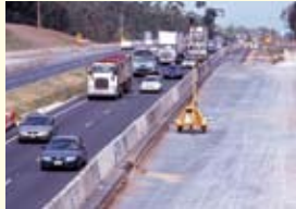
Bruce Highway upgrade
