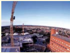
Prince Charles Hospital upgrade
